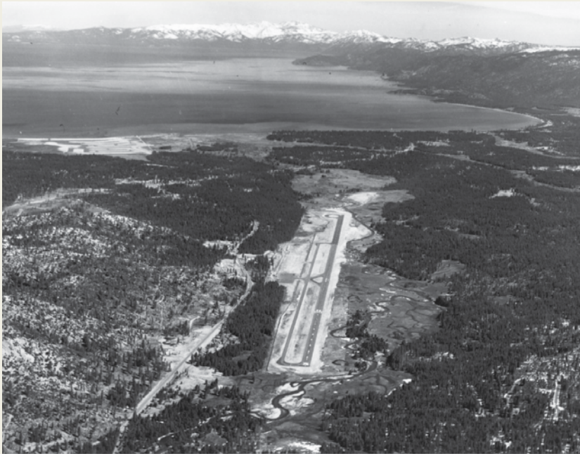
Airport Construction, 1960's
