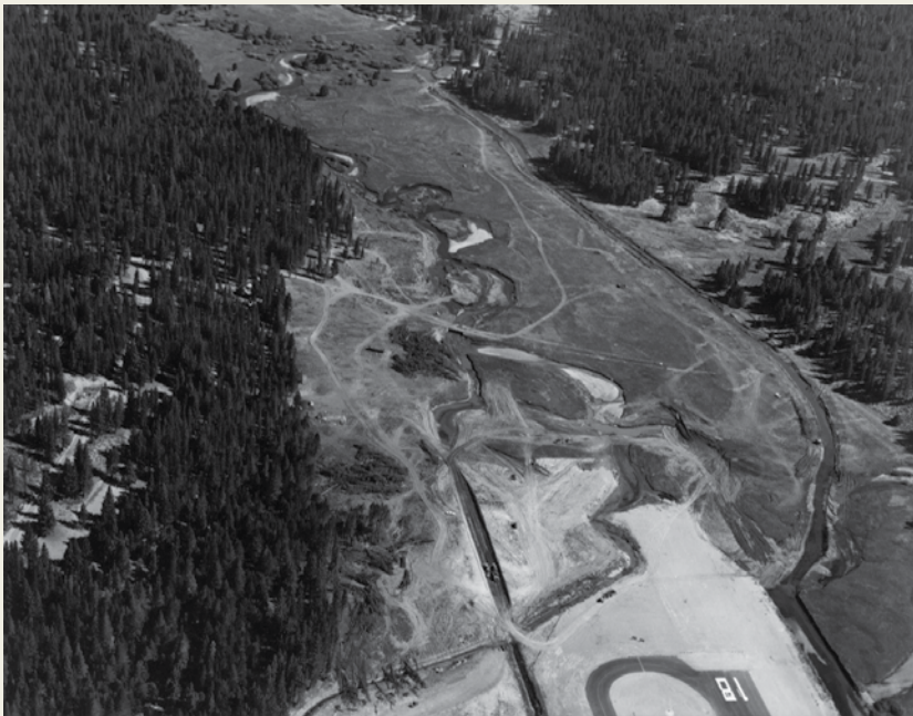
Airport Construction, 1960's
